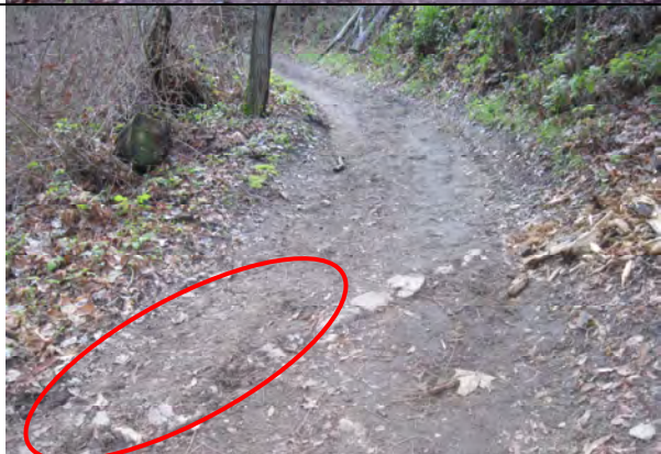
Top: A worn but otherwise good rolling grade dip is silting in; soon, water won't be able to leave the trail. Bottom: Drain on uphill side of an old rock waterbar needs cleaning out.
