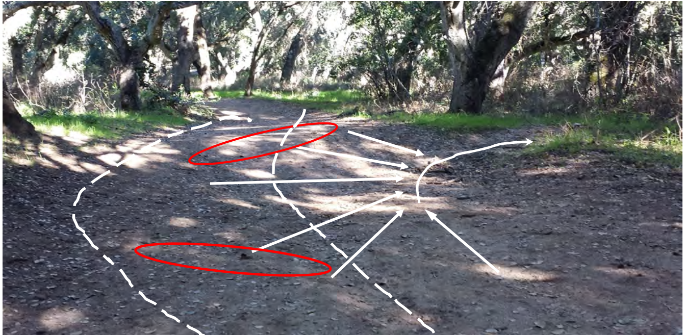
Seriously. Above: A long, wide Coweeta Dip. Hikers follow along the pathway (dashed lines), barely noticing the increased outslope (straight arrows). Water runs down the outslope and the outside edge of the trail, combining at the outer edge to flow off the trail (curved line). Sharp rims, circled in red , should be shaved down, for walking comfort. Known also as a “rolling grade dip” (see Early Autumn, 2014, TTN , p 3, for technical details).
