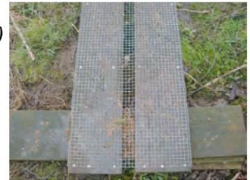
keep puncheon "floating" on the surface. Hardware cloth is bent around sides of stringers and fastened with staples or nails. Although called a 'cloth,' the material is actually metal – threads of hot-dipped galvanized steel "woven" into a mat of small squares (½" size squares recommended).
